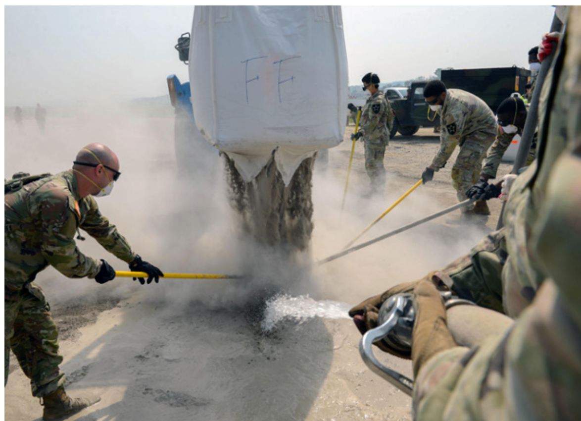
U.S. Soldiers assigned to the 11th Engineering Battalion and U.S. Airmen assigned to the 51st Civil Engineer Squadron mix flowable concrete fill during IRON RADR at Osan Air Base, Republic of Korea, April 24, 2025. The rapid airfield damage repair mission encompasses advanced pavement repair techniques and strategies that support airfield operations in degraded and contingency conditions, allowing swift restoration of combat airpower generation capabilities no matter the warfighting landscape. ▲
